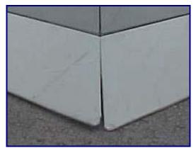
In so-called "Fisher-Price" parks—those constructed from modular, pre-fabricated sections—the geometry and quality of fit are often lacking.
