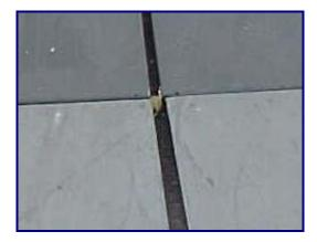
Thresholds that are separated and lifted off the ground present a danger to users of improperly constructed skateparks.
