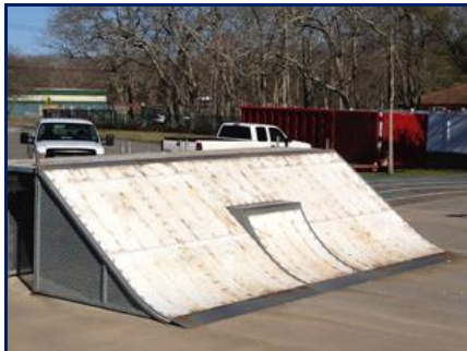
Existing ramp before repairs
