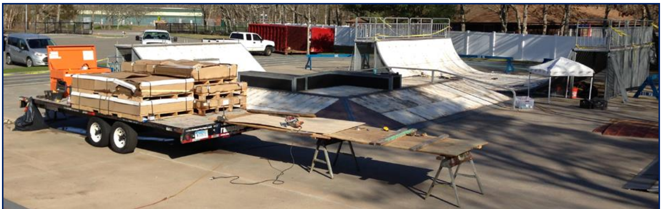
On-site Skatelite surface milling and installation
