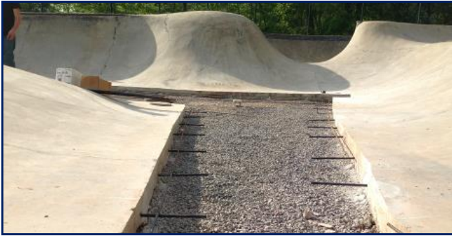
New drainage and sub-grade installed then placed and finished correctly
