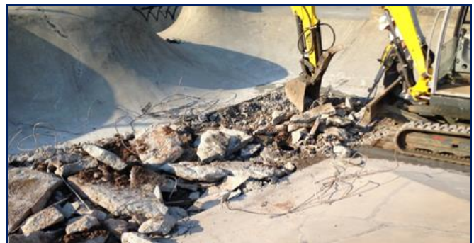
Bad concrete removed
