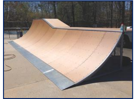
Repaired and resurfaced
