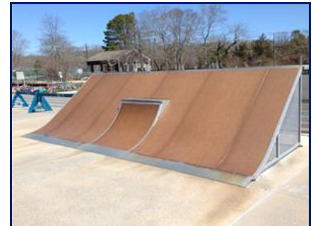
Repaired and resurfaced
